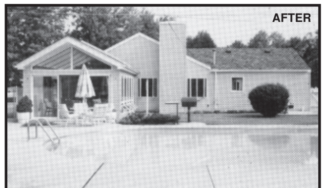
AFTER: New Roof System Offers Better Water Drainage and Updates Appearance Of The Home
